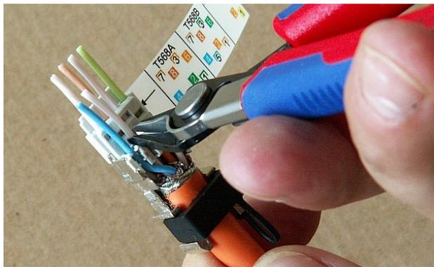
Fig. 5.55: Trimming conductors
