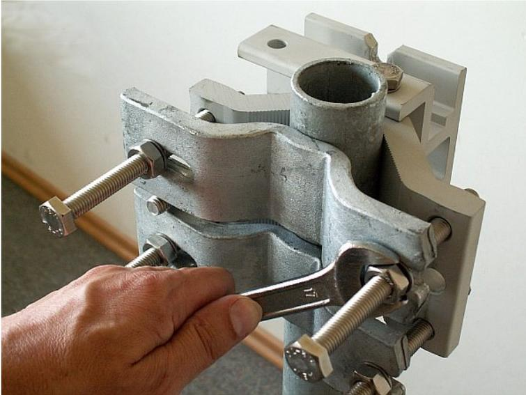
Fig. 5.7: Attaching the bracket to the mast tube
