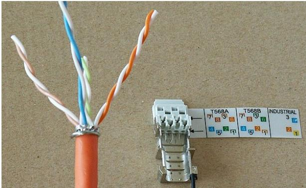
Fig. 5.51: Separated pairs of conductors
