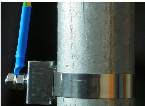
Fig. 5.66: Protective conductor at the mast on a ZSA16 terminal
