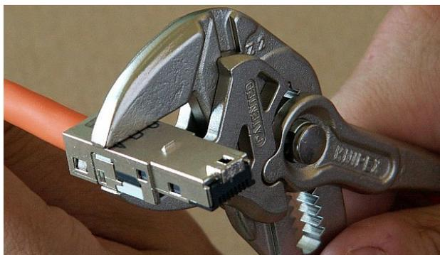
Fig. 5.42: Squeezing the connector until the locks snap into place
