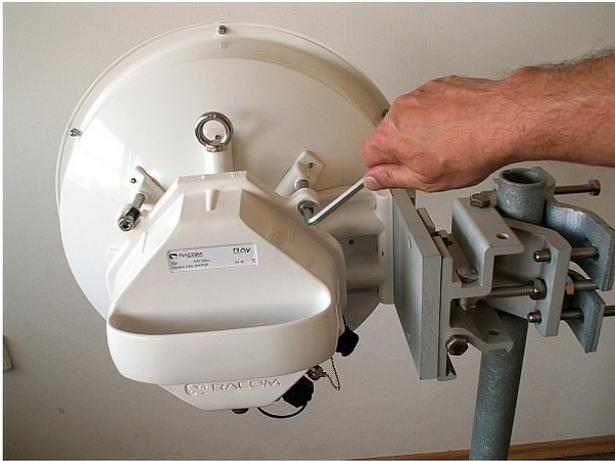
Fig. 5.15: Tightening bolts on the FOD unit
