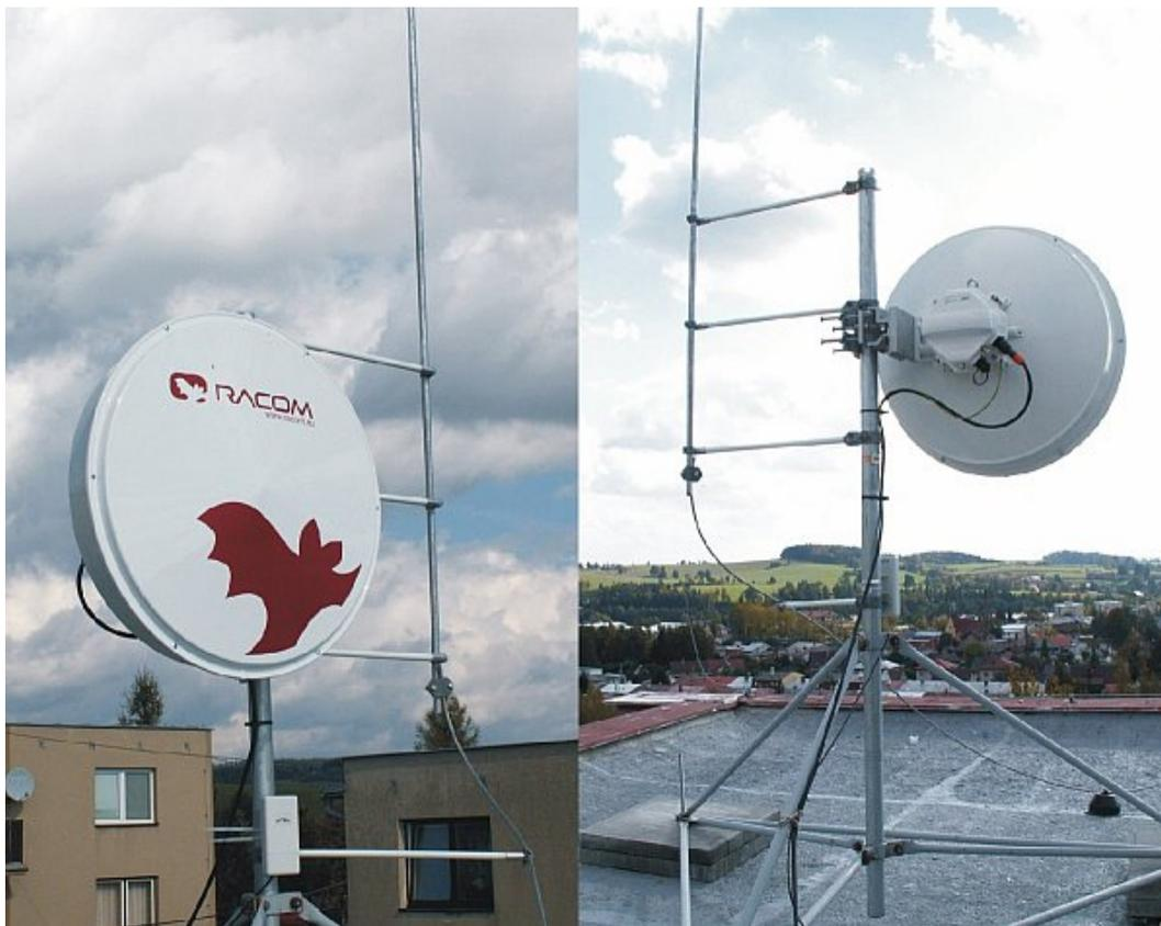
Fig. 5.67: Separated lightning conductor
