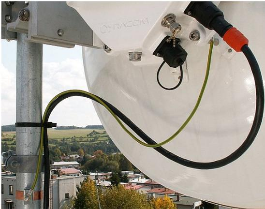
Fig. 5.64: Grounding the FOD unit
