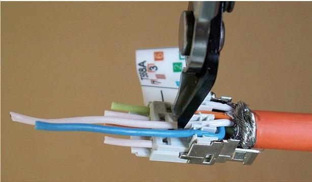
Remove the pinout sticker and fit the complementary half of the connector. Squeeze the parts together.
