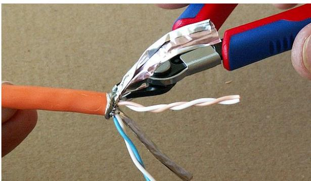
Fig. 5.50: Removing aluminium conductor shielding
