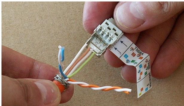
Fig. 5.37: Pushing the lower pairs into the connector
