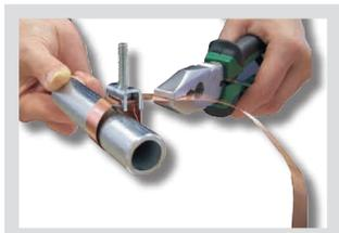
2. With the other end of the tape, wrap the pipe and pull through the insert according to the picture.
