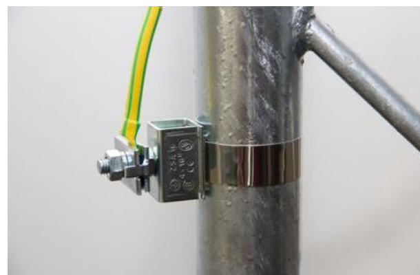
Fig. 4.10: Grounding the RAY unit
