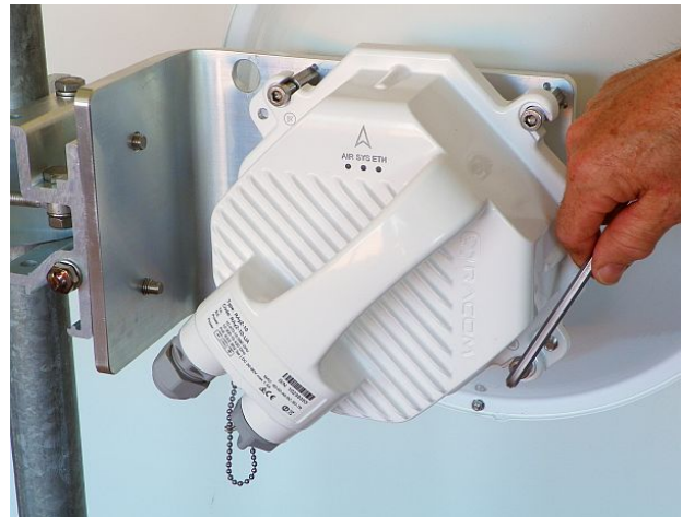
Fig. 17: Tightening bolts on the FOD unit
