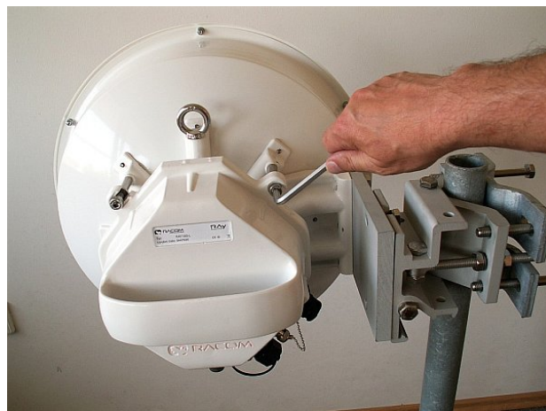
Fig. 5.15: Tightening bolts on the FOD unit
