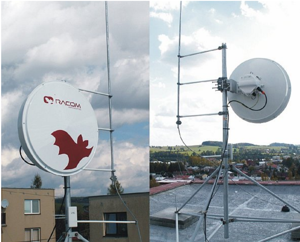
Fig. 5.69: Separated lightning conductor
