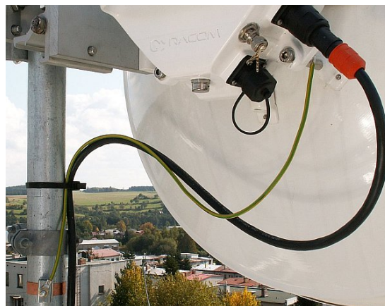
Fig. 5.66: Grounding the FOD unit
